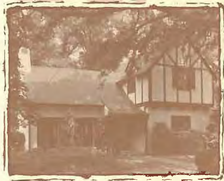
PERIOD REVIVAL Built in 1927, the Collin House at 1514 Cristobal Drive, is an example of Tudor Revival architecture. Note the half- timbering.
