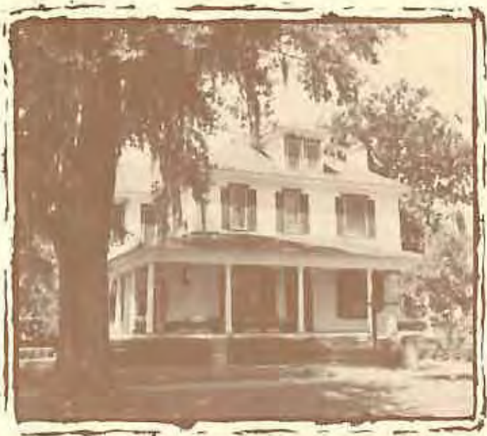
COLONIAL REVIVAL Built in 1906 at 318 North Calhoun Street, the Shine House is a basic pyramidal roof house with Colonial Revival detailing applied.
