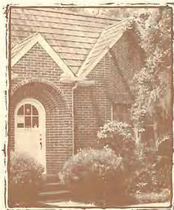
This building's unpainted masonry is an important character defining feature.
