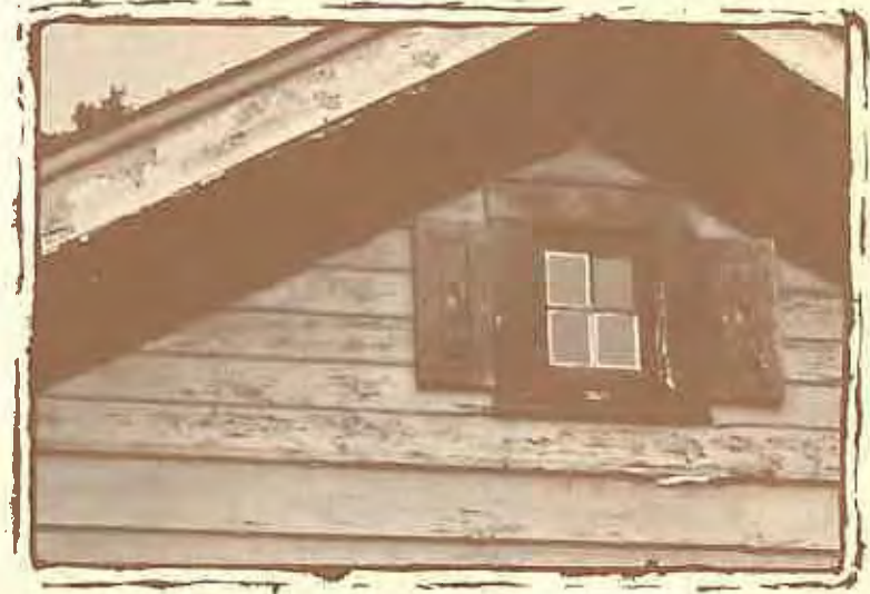
When preparing the building for painting, remove loose and damaged paint.
