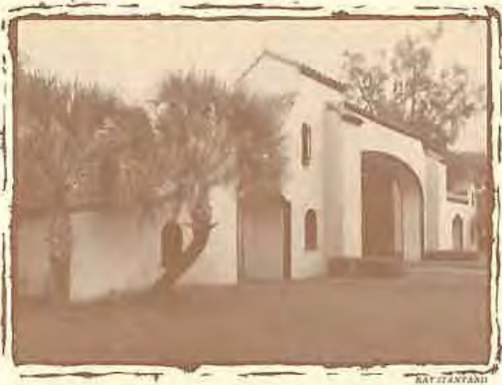
PERIOD REVIVAL The Los Robles Gate, with its barrel tile roof, use of arches, and stucco finish, is executed in the Mediterranean Revival style. It was constructed in 1927.
