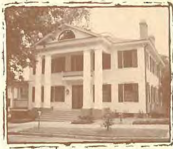
Although constructed in c. 1840, the Knott House at 301 East Park Avenue has been restored to its appearance in 1928, the year the Knott family acquired the house and made significant changes to the property.
