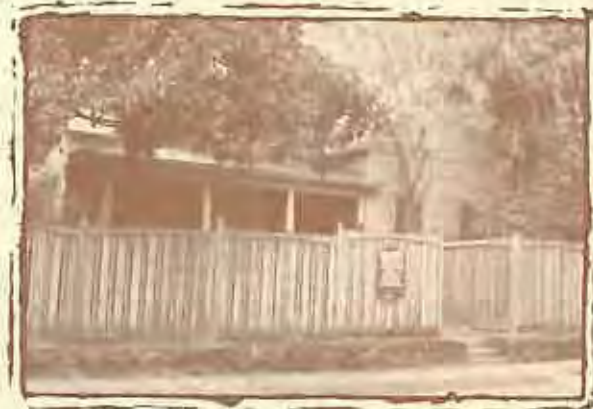
INAPPROPRIATE Although of wood, this fence is not transparent and is too high, blocking the view of the building from the district.
