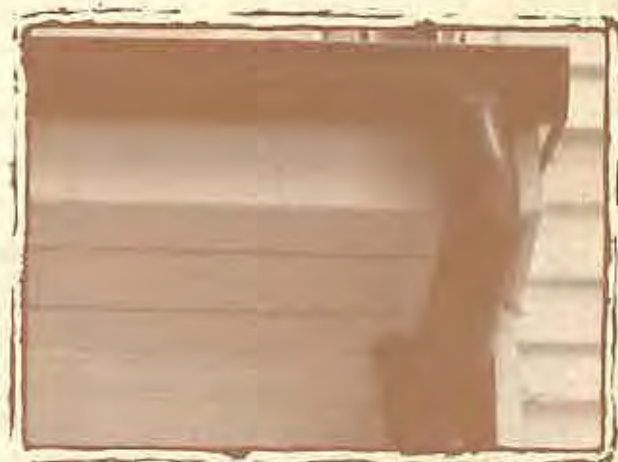
APPROPRIATE Copper downspouts have been used on the Knott House Museum.
