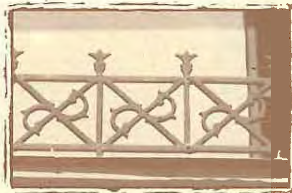
Details make historic buildings distinctive.
