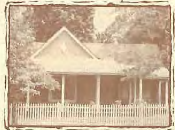
APPROPRIATE This non-historic fence illustrates the design elements of historic fences - it is approximately three feet in height and has a transparent quality.
