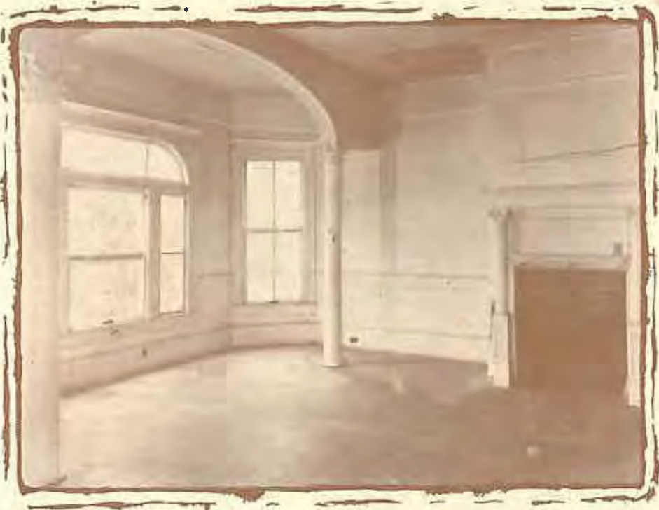
Interior changes such as dropped ceilings or permanent partitions that would alter the historic volume of this space are discouraged.
