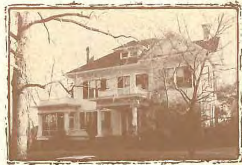
Constructed in 1913, the Lively House at 403 East Park Avenue contributes to the historic streetscape.
