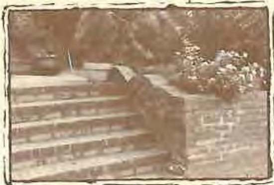
This brick retaining wall is compatible with the historic brick building.
