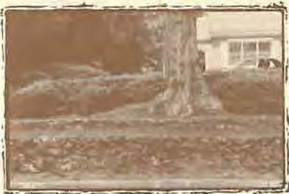
This rubble rock wall should be preserved.
