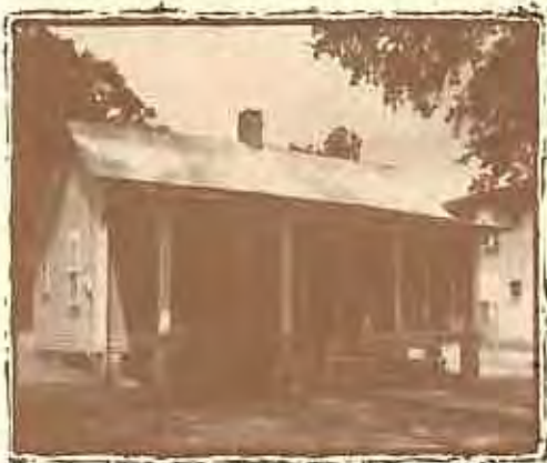
SIDE GABLE Built in c. 1910, this house at 444 West Carolina Street is an example of the one story side gable vernacular house. Note the similarity to Comte de Castelnau's 1838 illustration on page 5.
